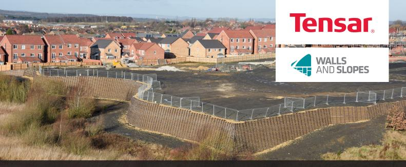
The TensarTech EcoCrib reinforced soil retaining wall increased the area of developable land on the former colliery.
