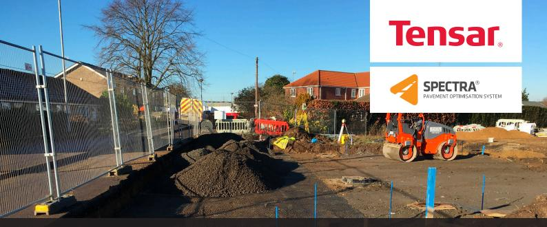
Ground conditions were highly variable, with the weakest soils having insufficient bearing capacity to carry the anticipated traffic loads.
