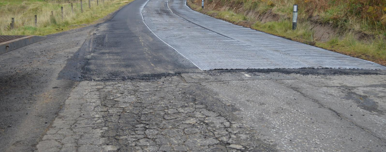
Tensor AX5-GN asphalt interlayer installed onto a 20mm regulating layer.
